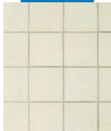
Grouting with colours matching the tiles
