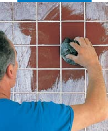
Final cleaning with a cloth
