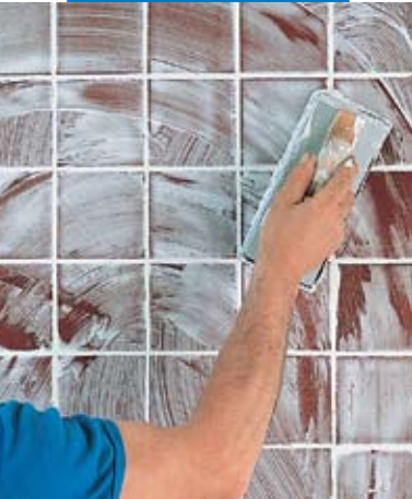
Spreading with a rubber float
